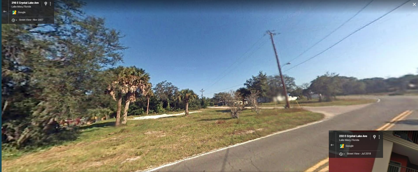
1st. St. and E. Crystal Lake Ave. November 2007 (Google Street View)
